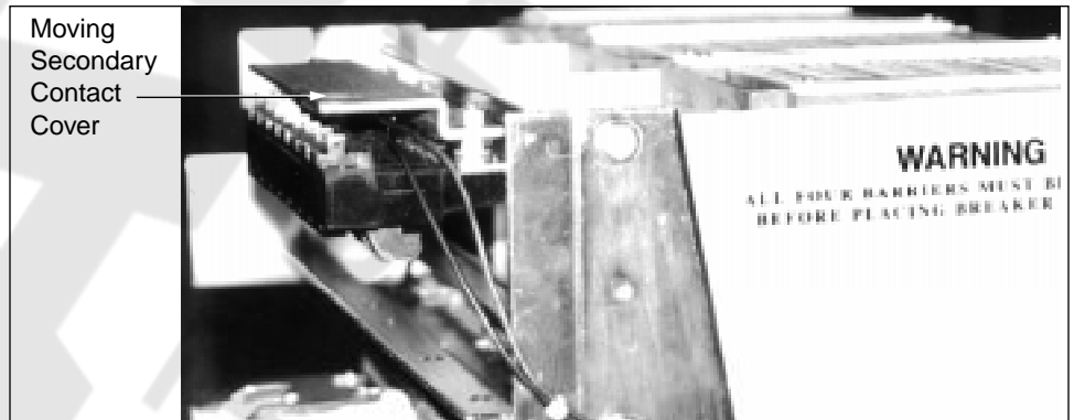
Figure 11: Moving secondary contact cover
