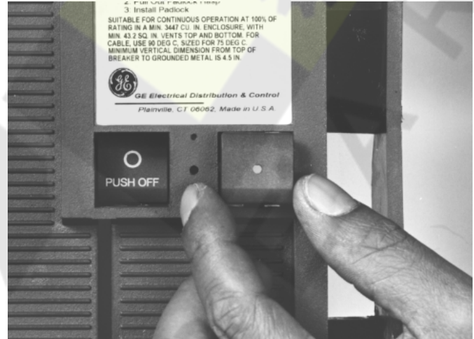
Figure 5. Installing the replacement On button into the breaker cover.
