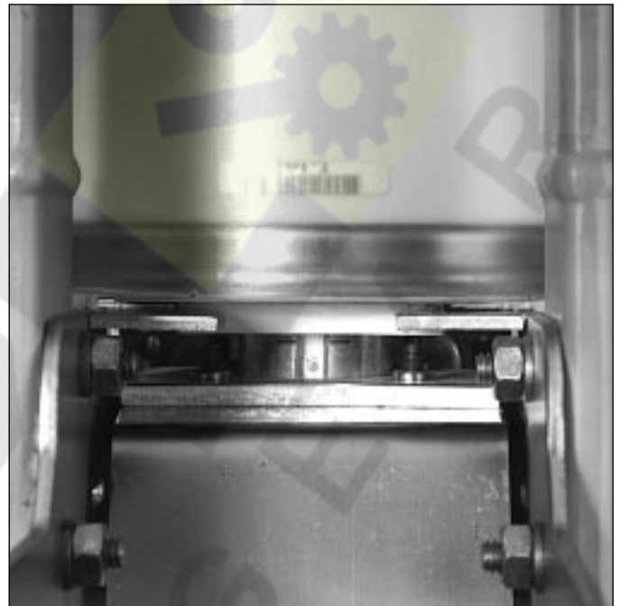
Figure 7-3 Vacuum Interrupter Showing Contact Erosion Indicator with Breaker Closed (Indicators are Checked Only When Breaker is Closed)
